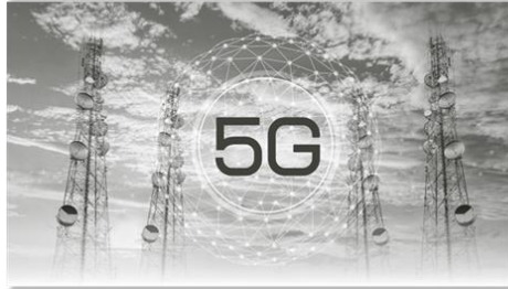
Open 5G Infrastructure
